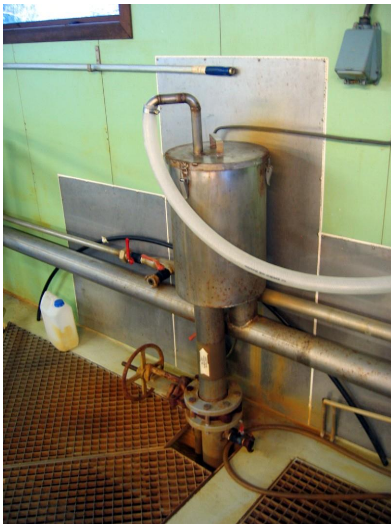
Figur 10 Mamutpumpe for sedimentering
