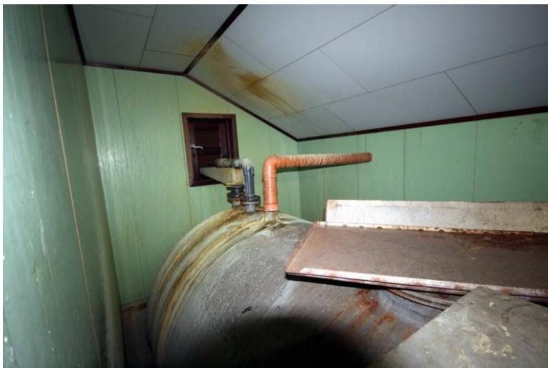
Figur 18 Tank for jernkloridsulfat
